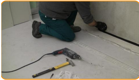
Lay the under wall strip
