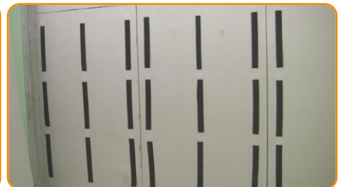
Apply Stywall S3A adhesive strip between each fixing
