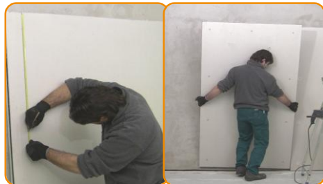
Mark fixing holes on each Mustwall 33B panel
