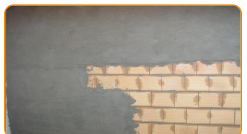
Realize the final plastering
