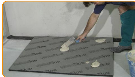
Apply the glue on the panel by spreading it on dots.
