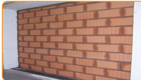
Build up the wall by caring to joint the blocks with mortar on both vertical and horizontal joints.
