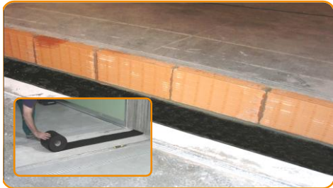
Lay the under wall strip in the dry floor before to build the wall.
