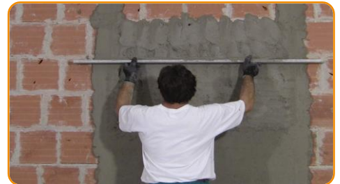
Apply in the first wall a layer of row mortar of about 1 cm thickness
