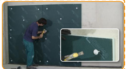
Apply the five plastic nails with the hammer.
