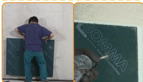
Place the panel on the right wall position and produce 5 holes per panel with the driller (one in the centre and one in the four corners)
